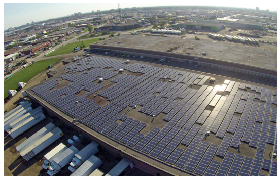
600 kW DC FIT 2 Project located in Brampton, Ontario.
